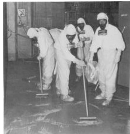
clean-up crew working to remove radioactive contamination at Three Mile Island.
