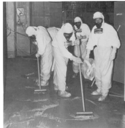
clean-up crew working to remove radioactive contamination at Three Mile Island.
