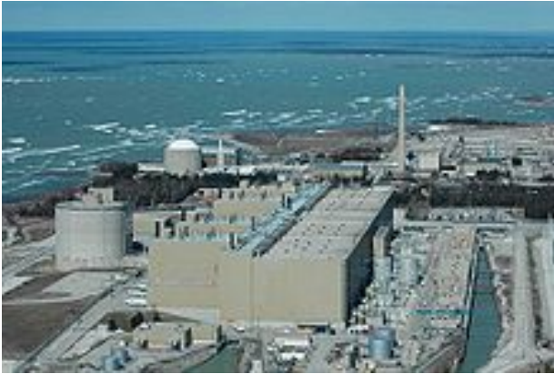
The CANDU Bruce Nuclear Generating Station in Canada is the largest nuclear power plant in the world. (900 MW)
