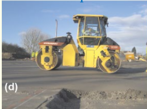
Placing and initial compaction of dry mix
