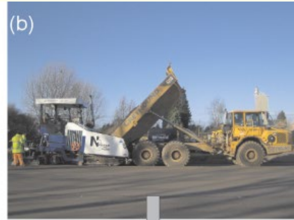
Placing of dry mix in asphalt pavement
