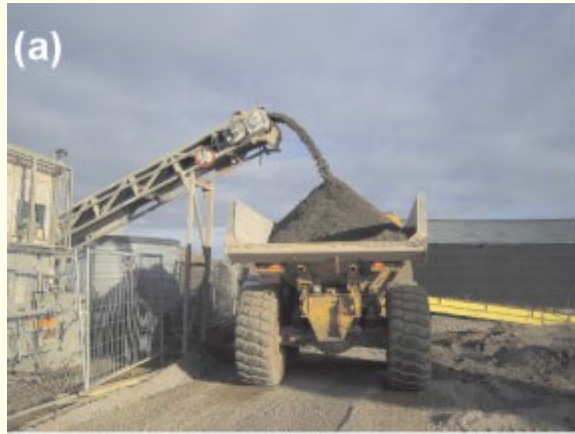
Placing of dry mix in truck
