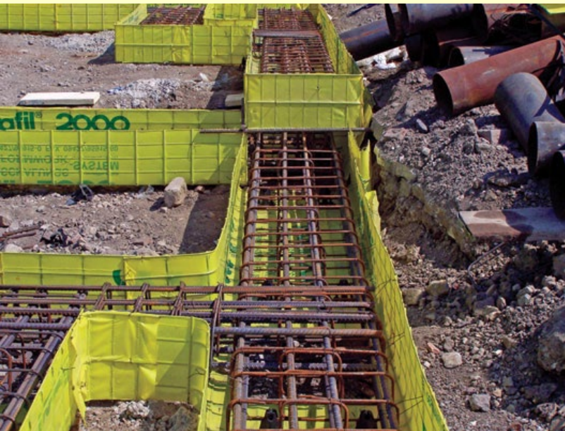
M & D foundations
